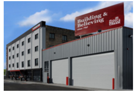
▲ Schweitzer, Inc.'s new office space and warehouse in downtown Battle Creek.
