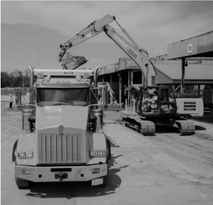
Pictured below: Parrish excavator loading a truck on a worksite
