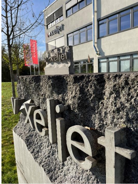
Sand mould printed and casted in concrete
