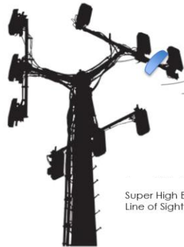
"Fiber Terminus" (on buildings or towers)
