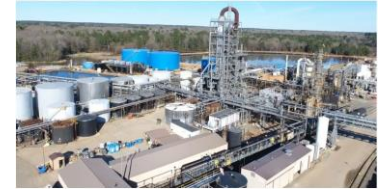
Smackover Refinery, Smackover, Arkansas
