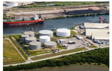
Asphalt and Fuel Oil Terminal, Tampa, Florida
