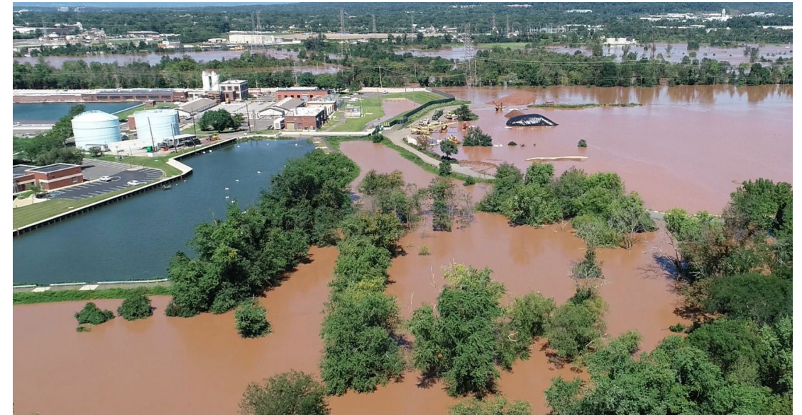
Raritan-Millstone Water Treatment Plant
