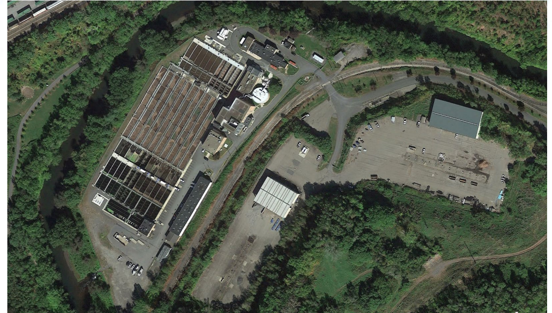
Aerial view of the former Scranton Sewer Authority and proximity to Lackawanna River
