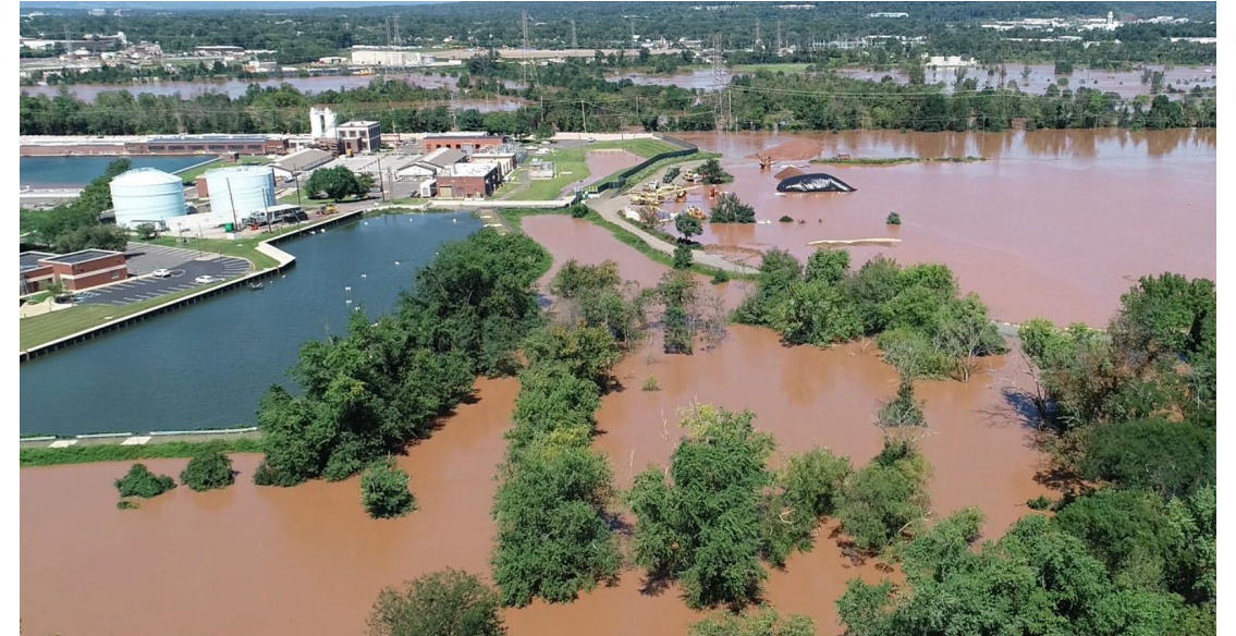
Raritan-Millstone Water Treatment Plant
