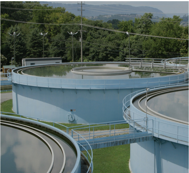
Aerial view of the Citico Water Treatment Plant in Chattanooga, Tennessee.
